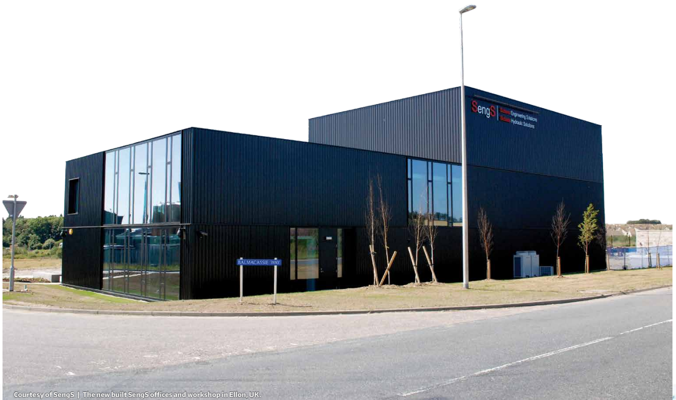
Courtesy of SengS | The new built SengS offices and workshop in Ellon, UK.
